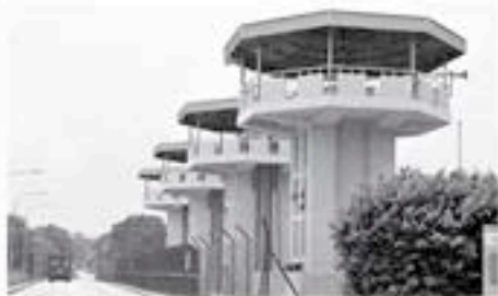
Tide Control - Kranji
