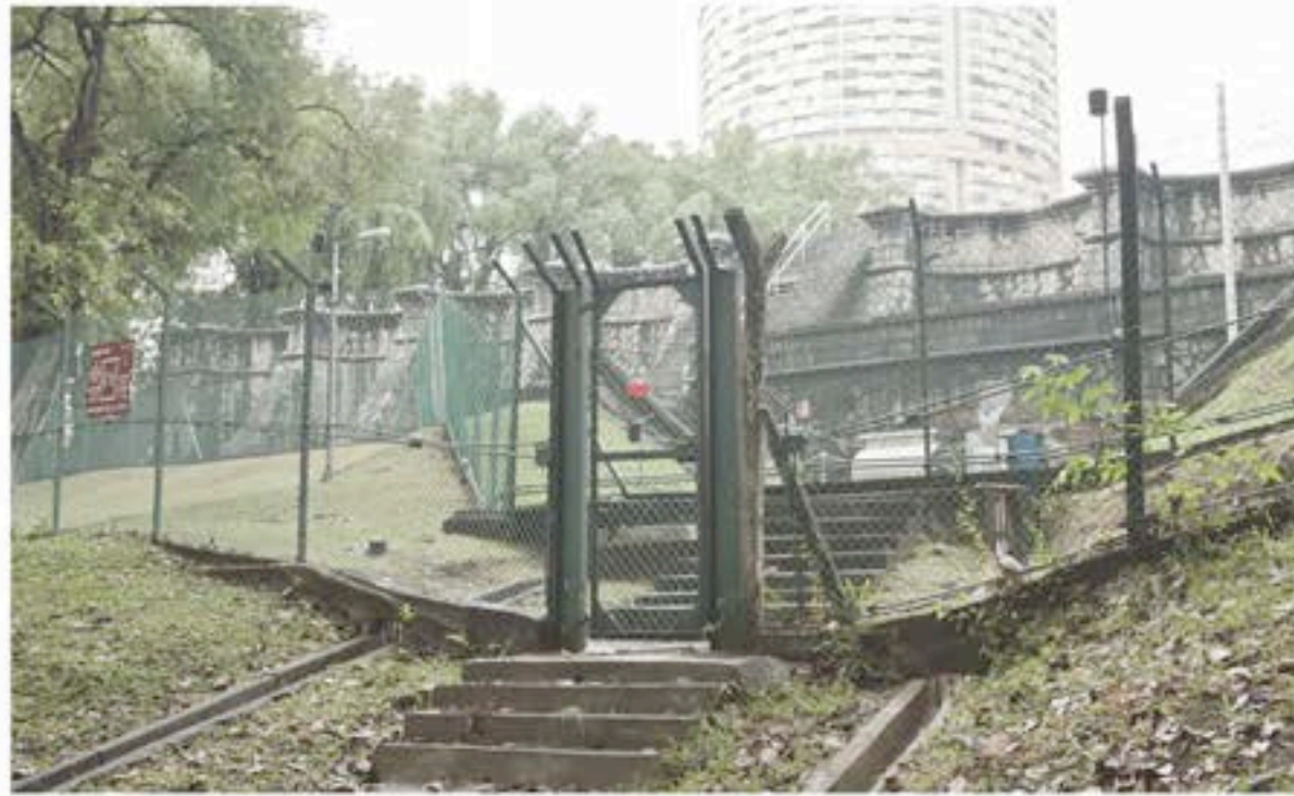
Fortress in CBD: Pearl's Hill Service Reservoir
