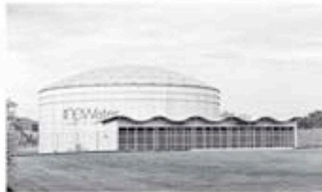
NEWater Plant - Changi
