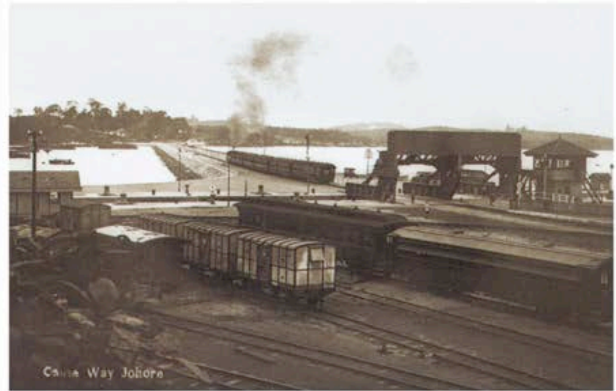
Causeway railroad in Johor Bahru
