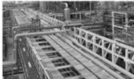
Left: Semboorp Pipeline
